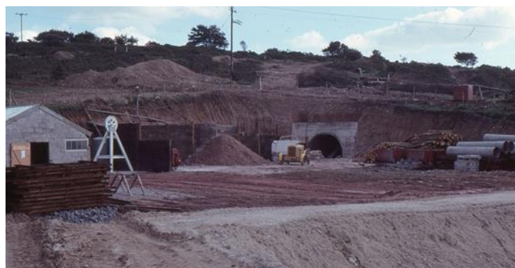
1985 AMAX Decline Portal, driving 70m underground into core of the resource
