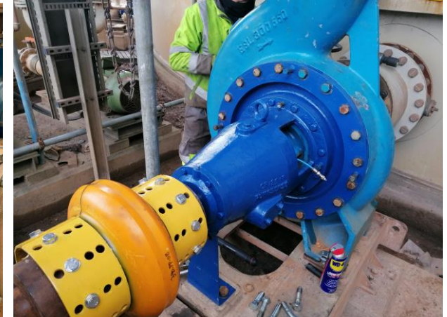
Pumps: inspection and replacement
