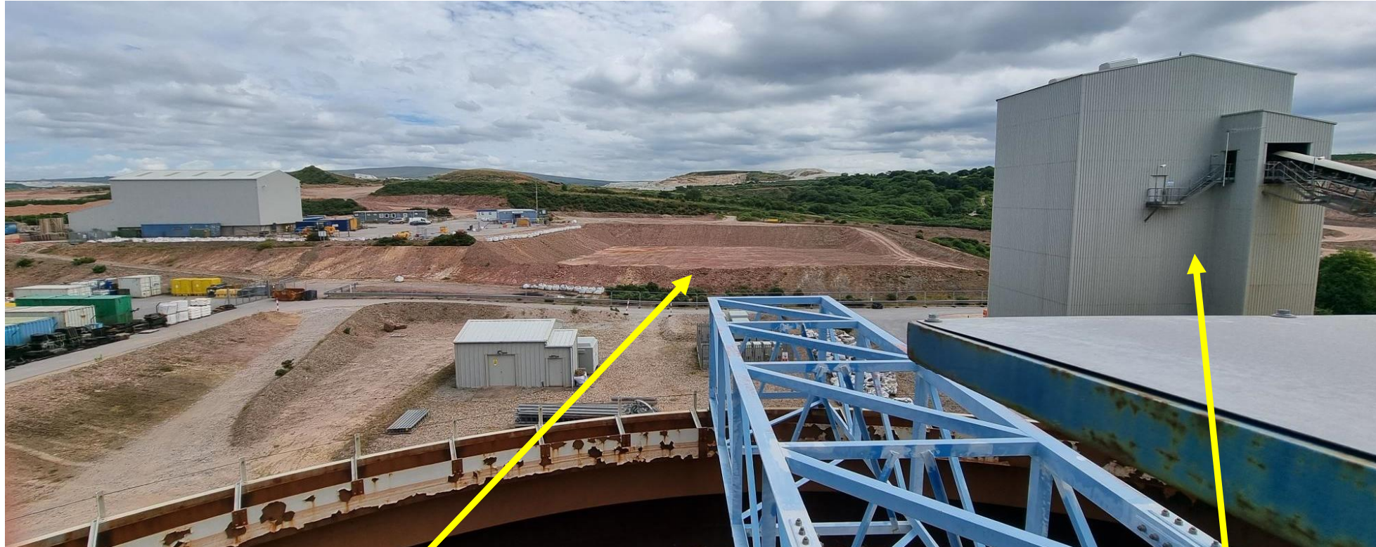
Ore sorter earthworks completed
