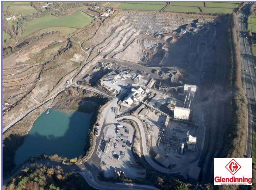
Above and right: CECA South West undertook a site visit to Linhay Quarry at Ashburton, courtesy of Glendinning
