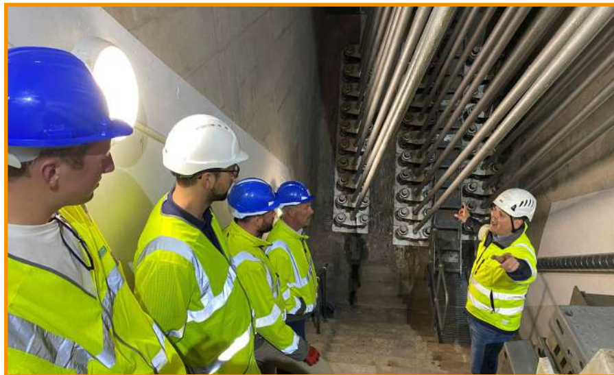
CECA SW site visit to Tamar Bridge in April where Richard Cole, Engineering Manager for Tamar Crossings, was our enthusiastic guide
