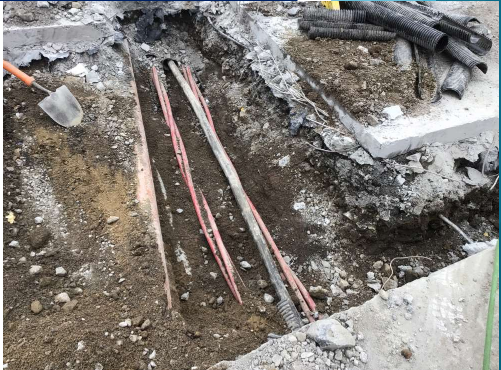
2 HV Cables, 1 LV Cable, Street light Cable, BT duct and drain pipe under reinforced concrete
