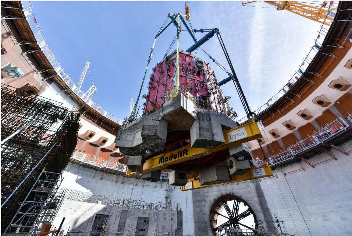
Reactor Cavity Pool lift 700 tonnes
