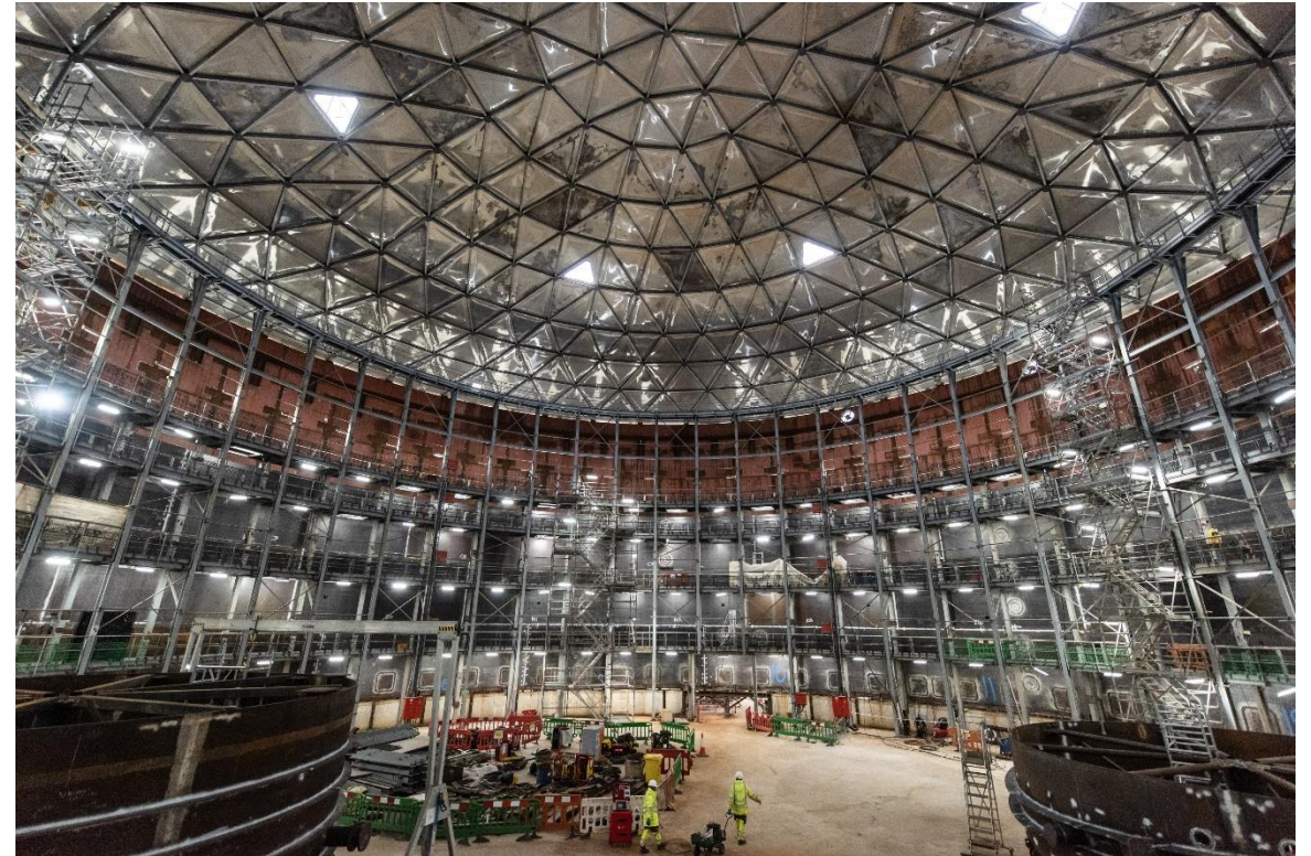
Bunker factory – for liner rings and domes
