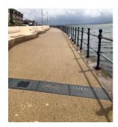
The scheme is 1km long, with a 1.2m high sea wall (resembling a wave), and will protect 70 properties at risk of flooding now from extreme tidal events, and give more than 500 properties improved protection over the next century.
