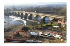
Over 200 cubic metres of low-carbon concrete has been poured to construct the Matlock flood wall, with approximately 8 tonnes of steel reinforcement.
