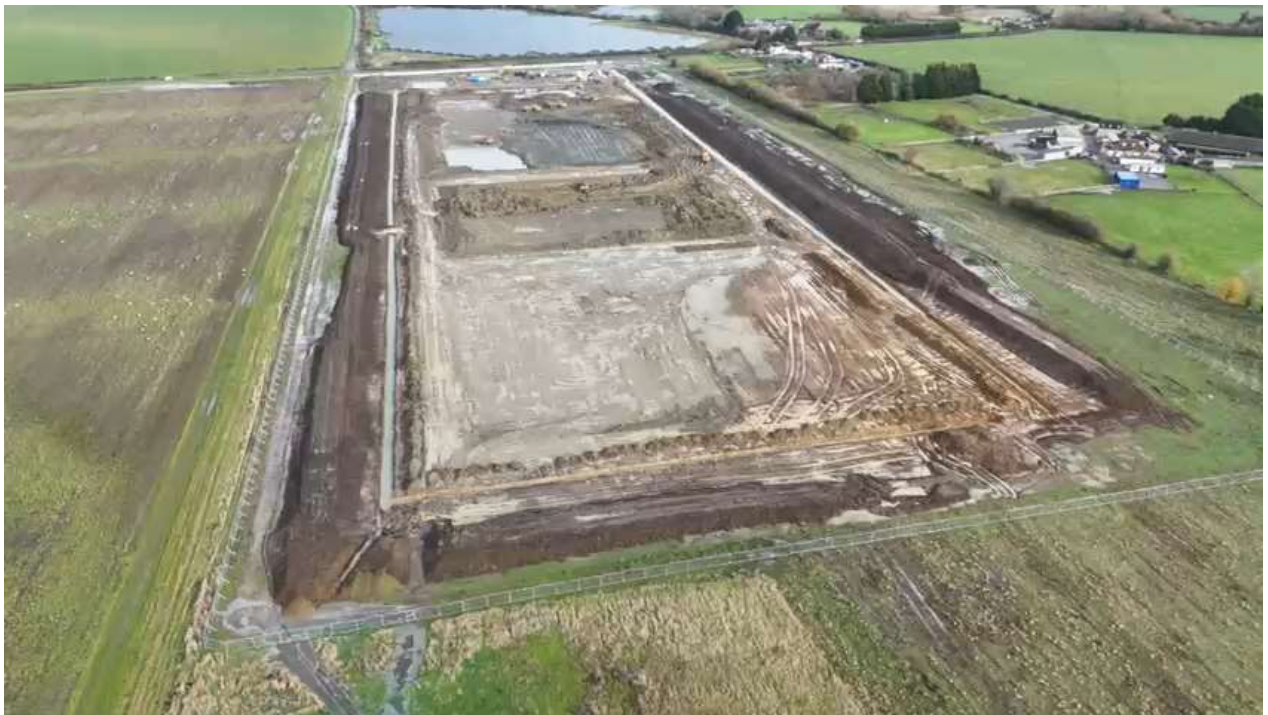
Figure 2 - SESRO Clay Compaction Trial site
