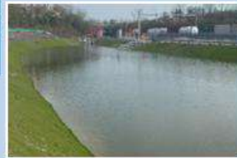
Example of lagoon at Chipping Sodbury
