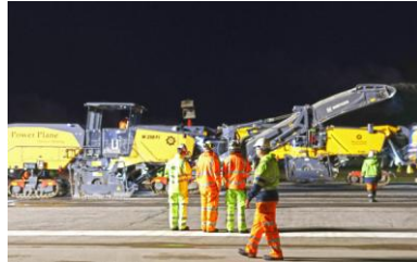
Airfield improvements including new Rapid Exit Taxiways
