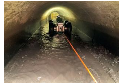
CCTV EXAMINATIONS, CULVERT JETTING
