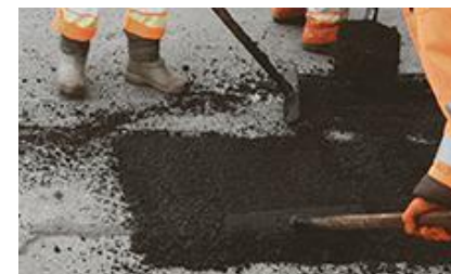
SURFACE REPAIRS AND CIVIL WORKS AROUND STATIONS AND DEPOTS
