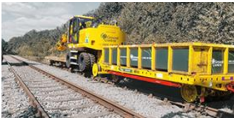
ROAD TO RAIL (RRV) ON-TRACK OPERATIONS
