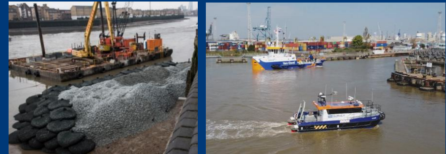
Dredging and river works
